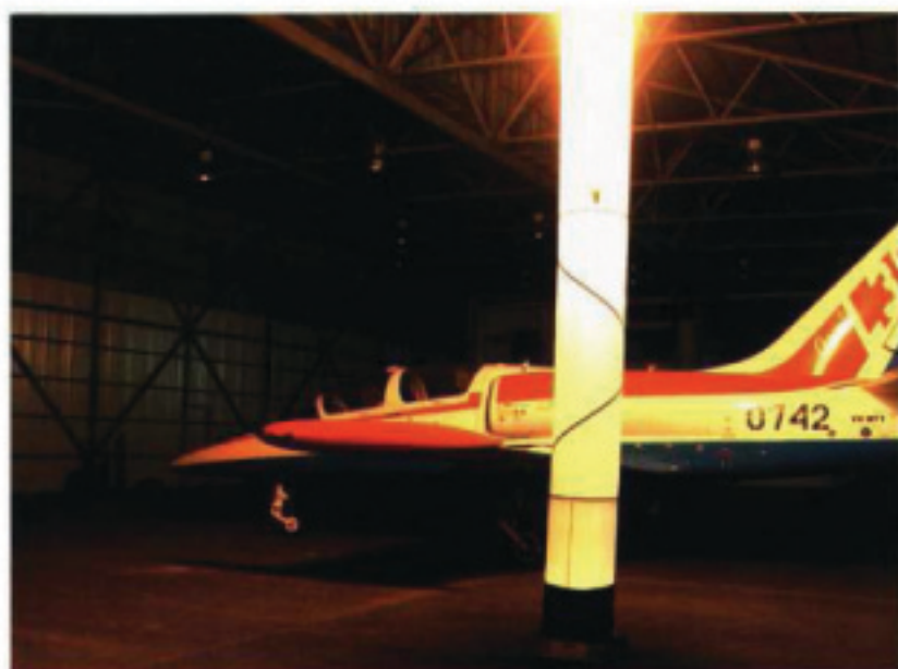
Shadows that normally accompany flood lights are greatly reduced and as the tower is lit from above.
